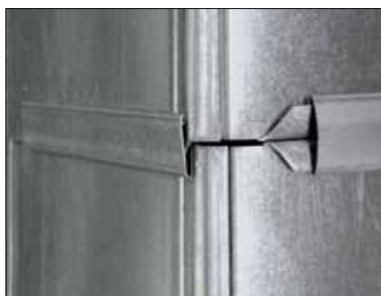
„S“ seam and drive cleat
