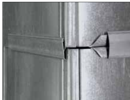
„S“ seam and drive cleat
